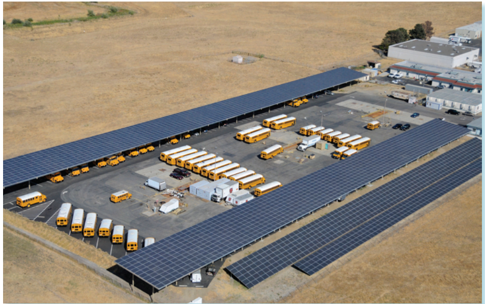
The innovative solar PV system at Solano County incorporates a ground-mounted solar array and dual-purpose solar bus-ports that shade the County’s school buses while generating powerful clean energy.
